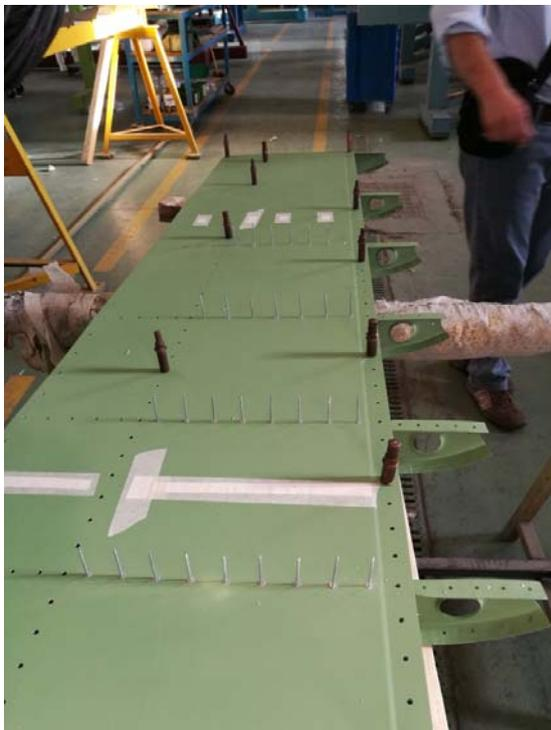
Figure 47 – Lower skin riveted on the wing box ribs
