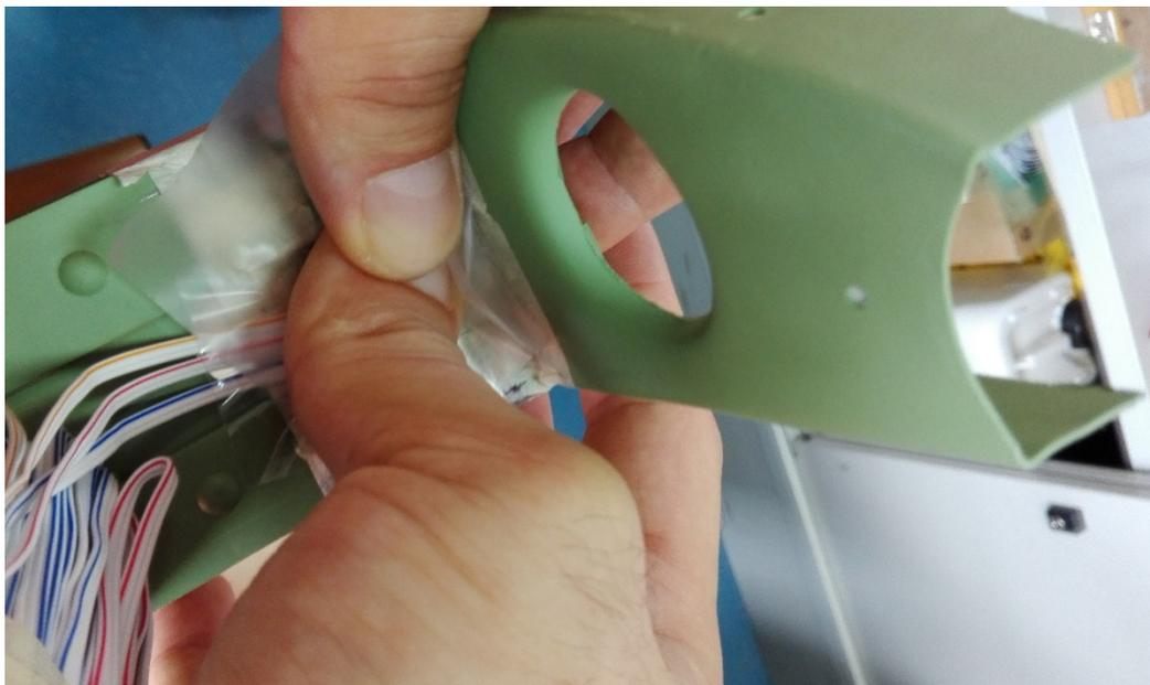
Figure 35 – Hand pressing for the adhesive bonding of the SG on the surface
